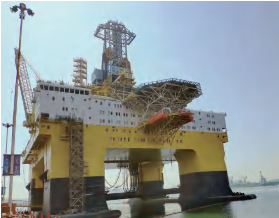
Figure 5 Construction Drilling Platform Blue Whale II
