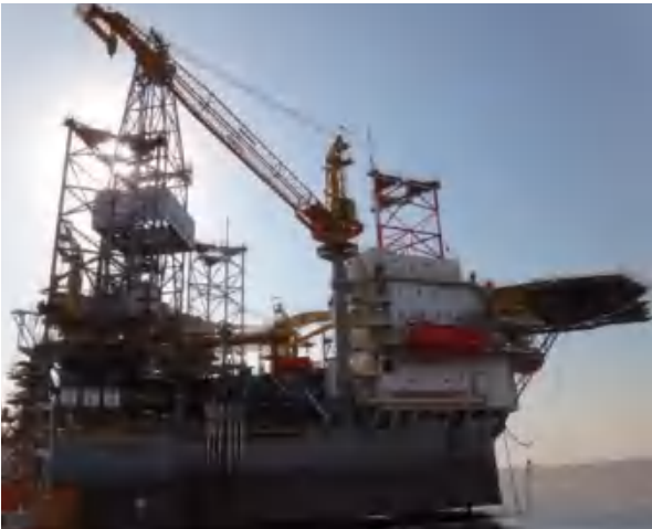
JU2000E Platform After Penetrating Legs (By SWS)
